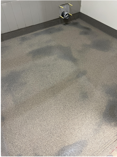
Installing resinous flooring on level 2.
