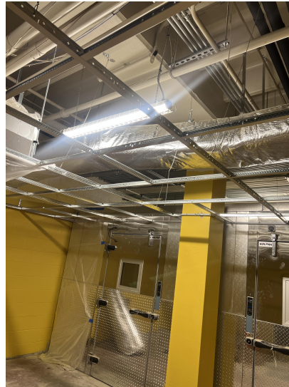
Installing ceiling frames in cooler freezer room on level 1.
